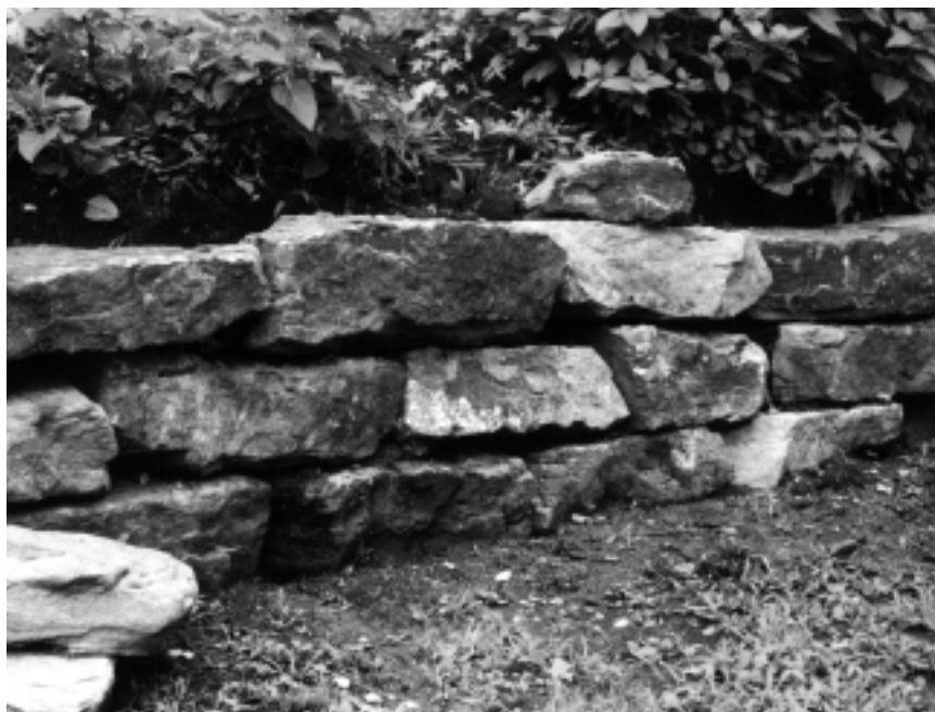
Staggered joints will result in a more solid and longer lasting wall.
