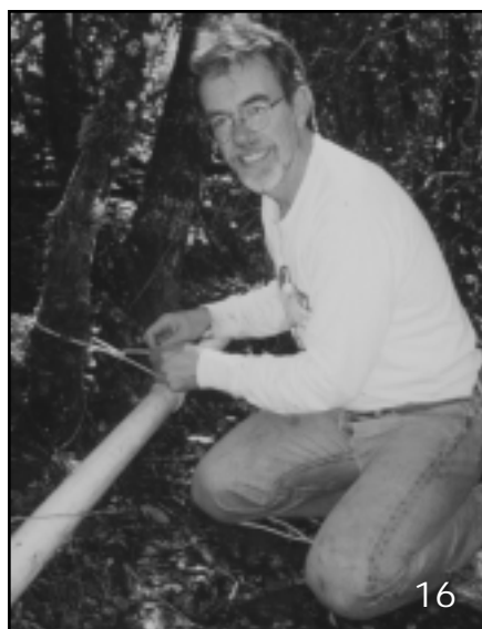
16. The pipe track is secured every 10-15 feet with nylon rope. Don't bind it tight to the anchor point.
