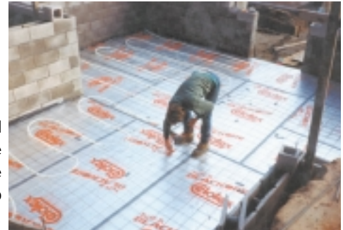
Right: Foam insulation and wire mesh are added. The hydronic heat pipes were tied to the mesh prior to the pour of concrete.
