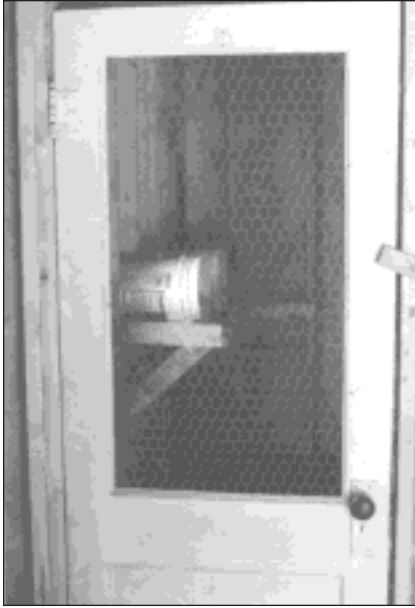
"Screen door" made by cutting out wood panel and adding chicken wire.
