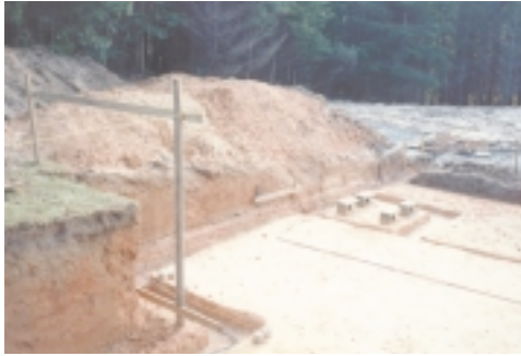
Left: The top soil from the building site was carefully separated and saved for a garden site
