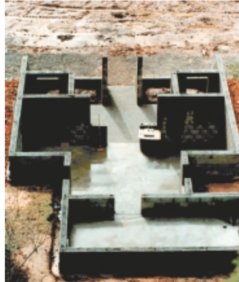
Left, above, & right: The foundation for the tower serves as structural and thermal mass and provides 300 square feet of comfortable living space.
