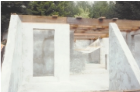
Left, above, & right: The foundation for the tower serves as structural and thermal mass and provides 300 square feet of comfortable living space.
