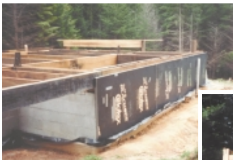
Above: The entire outside of the house is wrapped in an insulating envelope.
