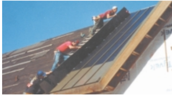
Left: A Uni-Solar module is lifted to the roof and installed.
