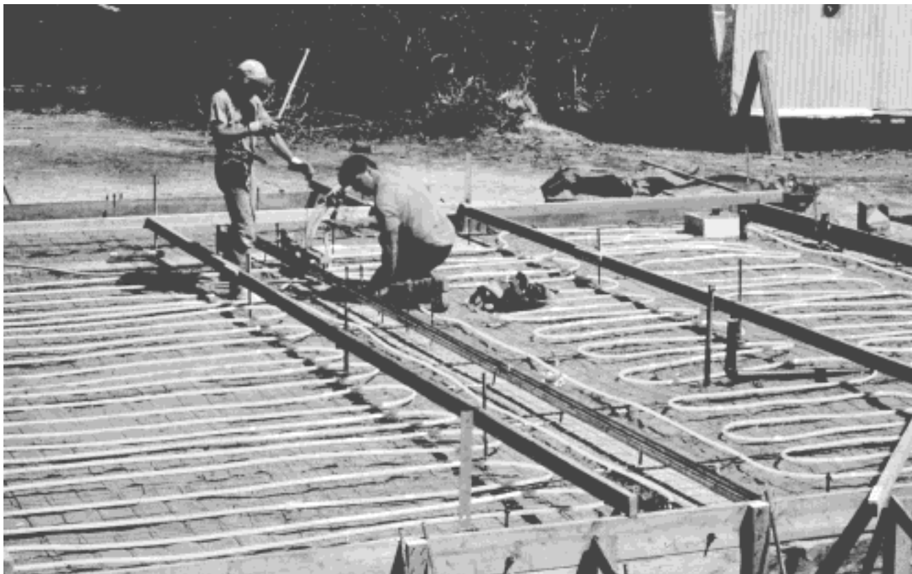
The McMillan foundation is inlaid with insulation and tubing and checked for leaks prior to pouring the slab.
