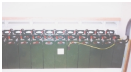
Below: Most battery packs use deep-cycle, lead-acid batteries.
